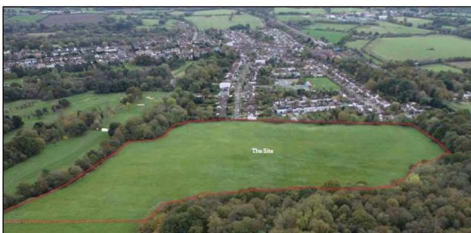
Figure 2.1: Looking south over the appeal site and Brookmans Park beyond.
